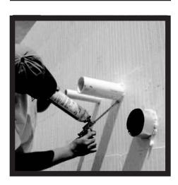
Identify and size all service and utility penetrations. Install all appropriate and properly sized sleeves where required. Keep in mind that lightweight sleeves can be crushed during concrete placement.
