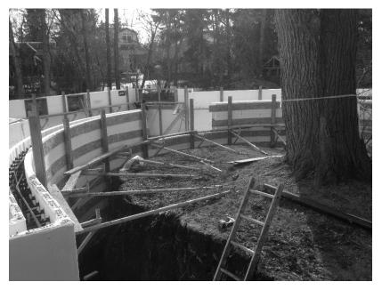
Foam adhesive can be used on wood and plastic bucks to provide additional buck support.
